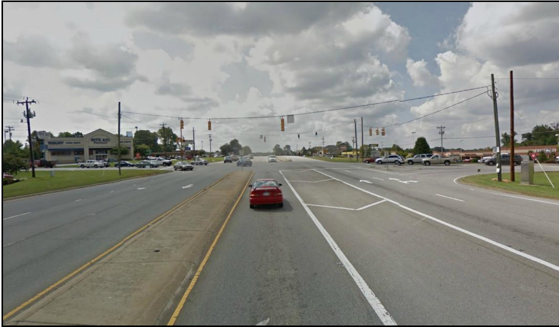
Google Maps (September 2012) – Looking South on NC 150 Approach
